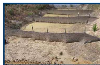
Temporary Rock Sediment Dam, Type B 1634.02
