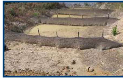
Temporary Rock Sediment Dam, Type B
