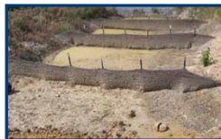
Temporary Rock Sediment Dam, Type B 1634.02 53
