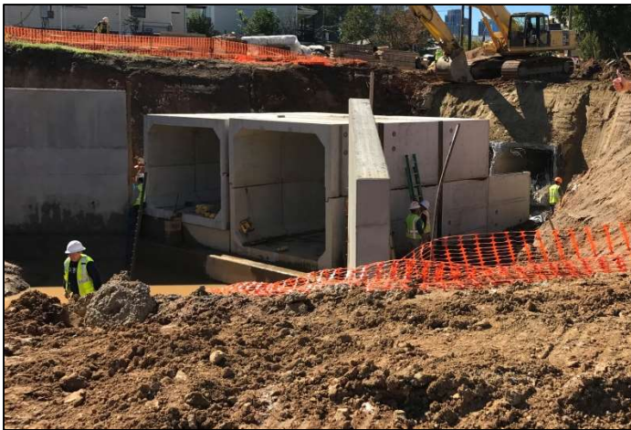
Maintain storm water infrastructure
