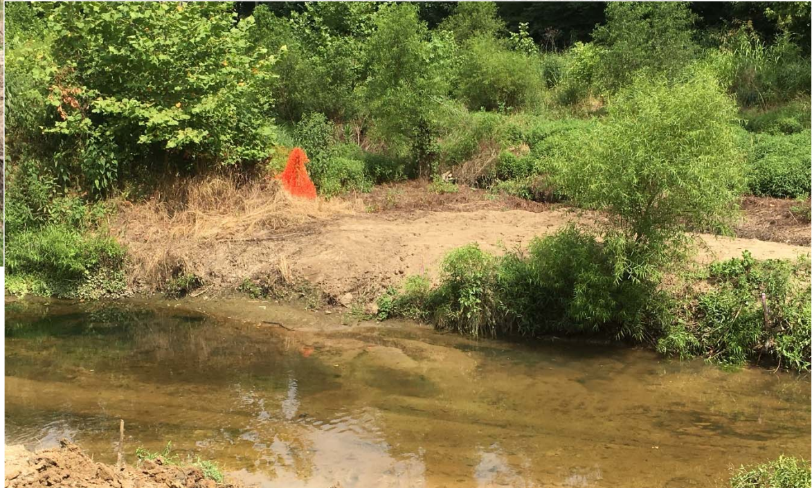
Immediately after repair
