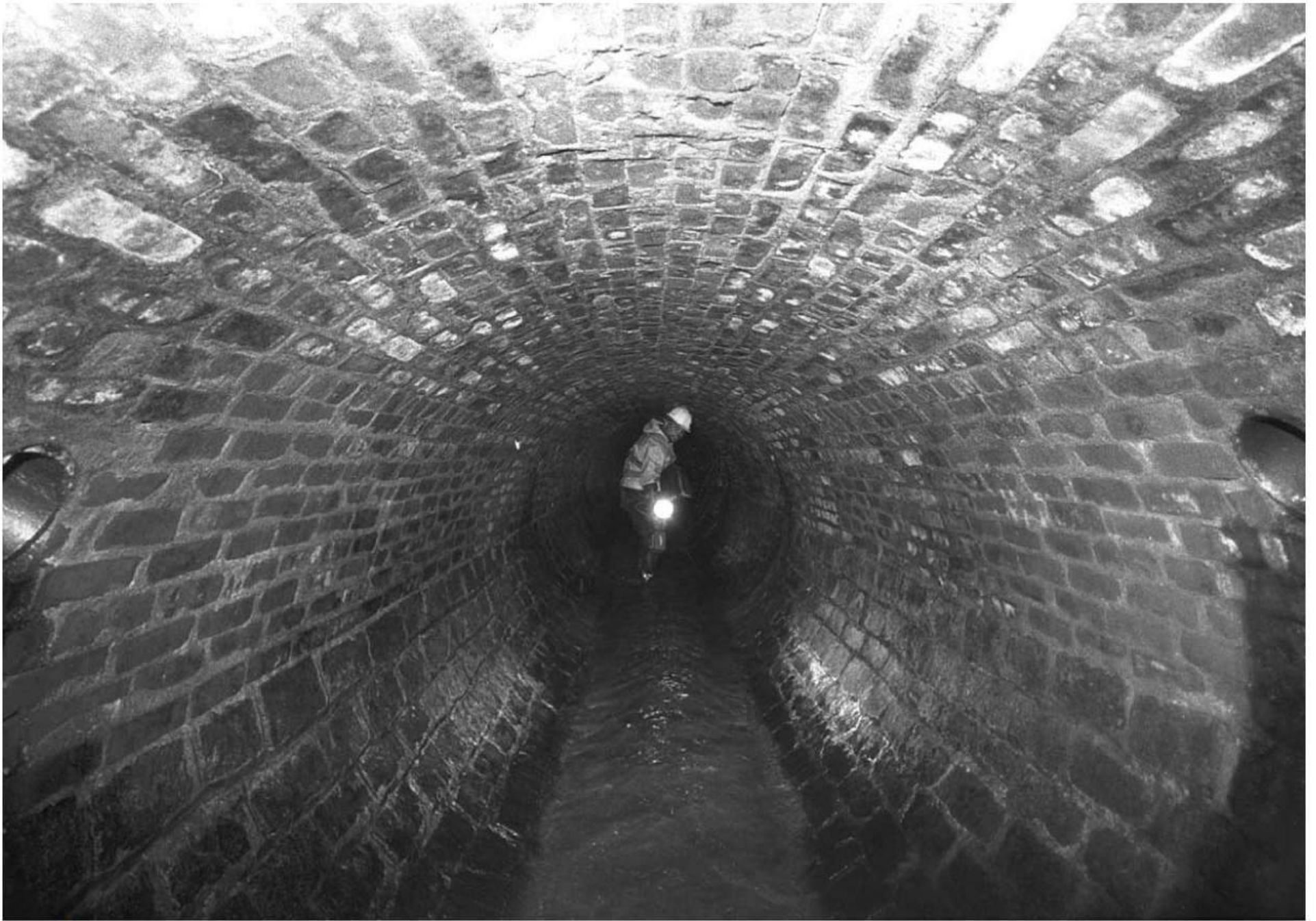
Brick sewer from the 1800s
