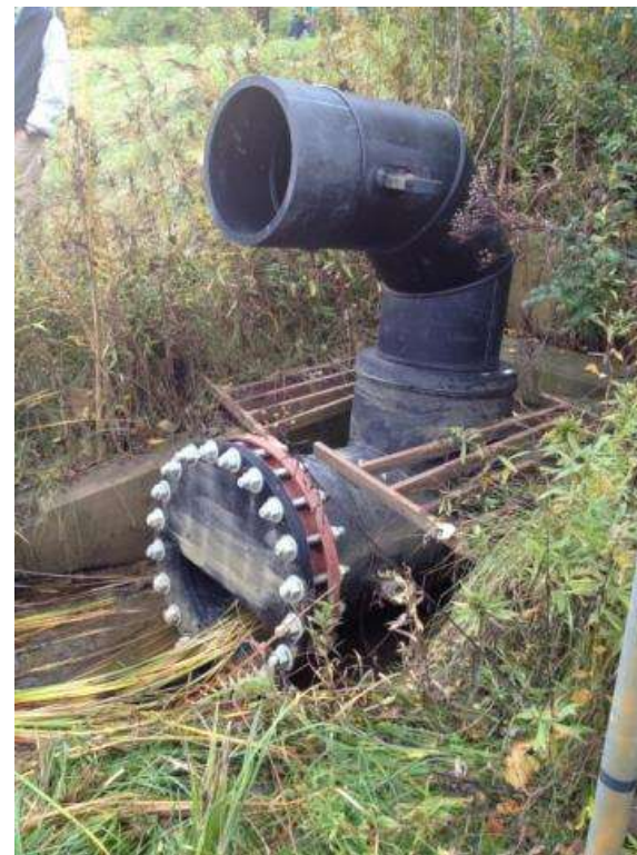
RESTRICTED OUTLET WITH BYPASS
