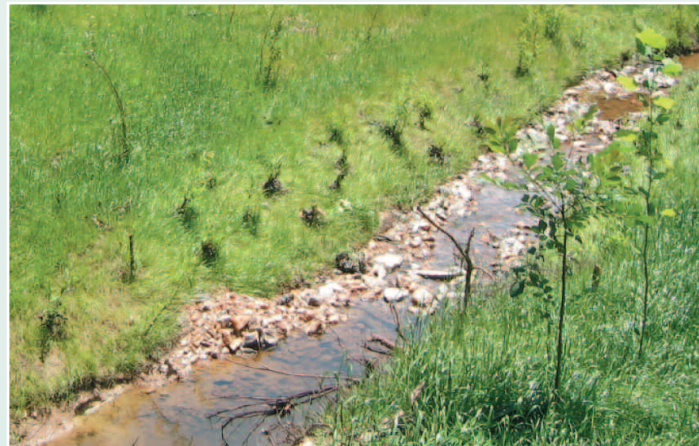
The same backyard stream six months after construction. With new plants and a new shape for the stream bank, the stream is much less prone to erosion. Young sycamore and birch trees and willow shrubs will create a shady, attractive space as they grow.
