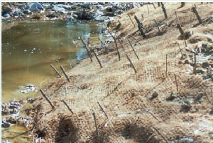
A backyard stream under construction. Erosion control matting covers the bare surfaces. Live stakes (cut from the willow trees) will grow into new shrubs.
