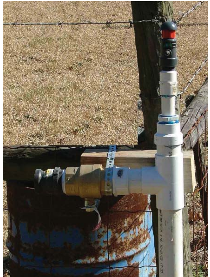
Figure 1. Regular flushing using a flushing riser assembly as shown here is important to prevent emitter clogging.
