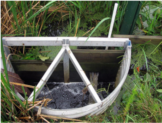
Figure 9. An outlet employing the traditional flashboard riser
