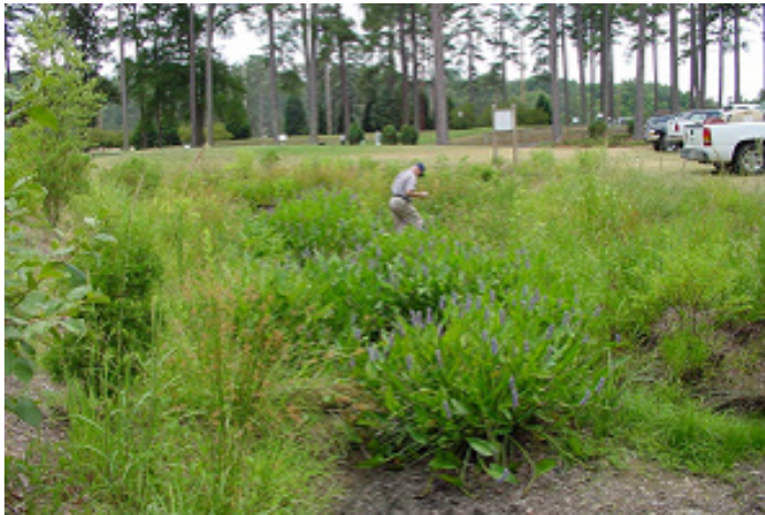
Figure 5. A stormwater wetland in Durham during the drought of 2002. Note the pickerelweed (a plant that usually flourishes in 3 to 6 inches of water) that is “high and dry.”
