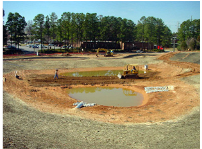
Figure 7. Topsoil being replaced on the wetland fringe of a wet pond
