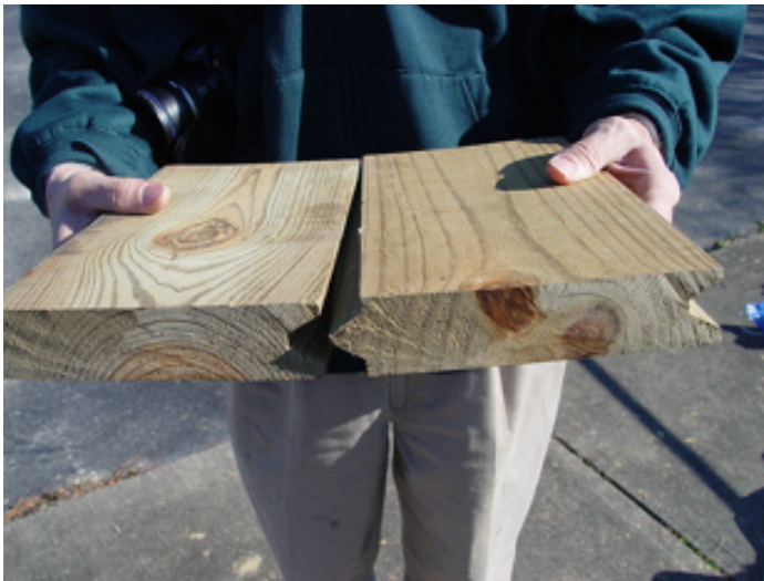
Figure 10. Small flashboard riser boards are stacked tongue-in-groove.
