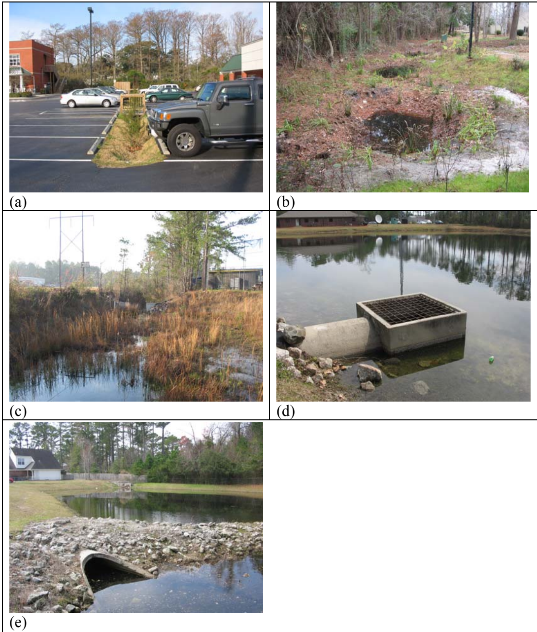
Figure 2 – Illustrations of BMPs: Port City Java Bioretention (a), Stonestrow Stormwater Wetland (b), Laney High School Stormwater Wetland (c), Cinema Wet Pond (d), and Residential Wet Pond (e)
