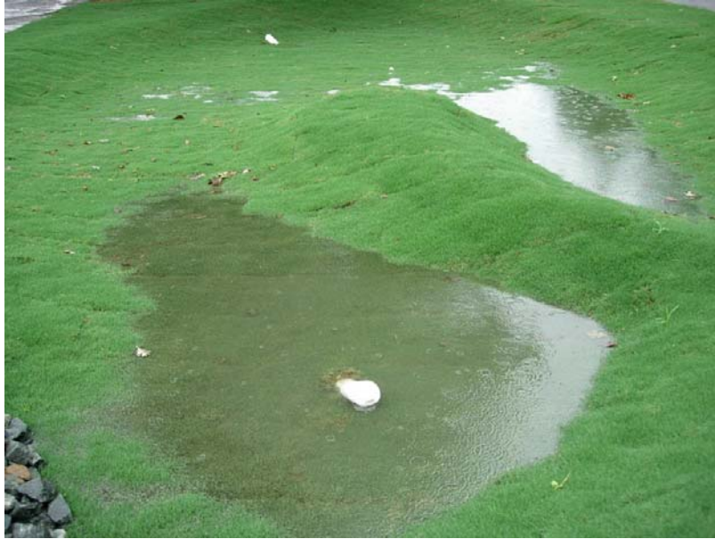
Figure 1. Grassed bioretention cell during a rain event.
