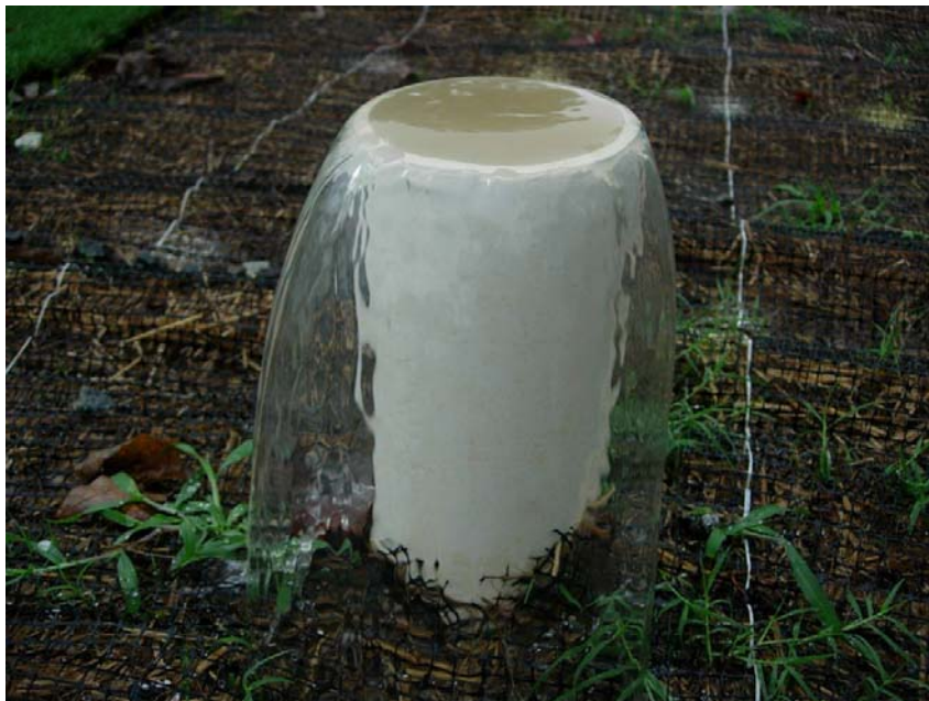
Figure 3. The upturned elbow flowing during a storm event. This designed allowed for more water capture and infiltration to the in situ soil.
