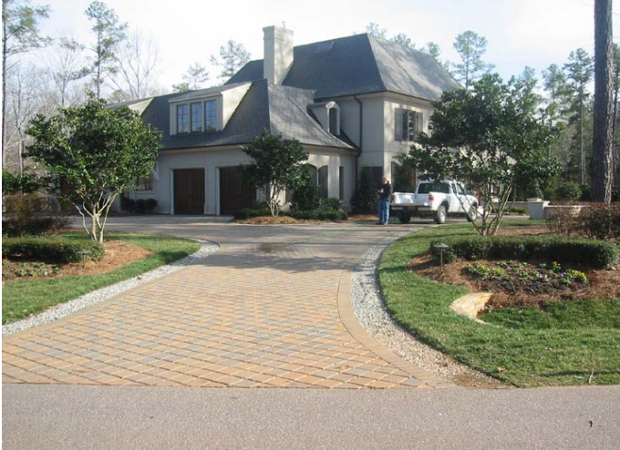
Figure 2. Cary PICP water quality monitoring site.
