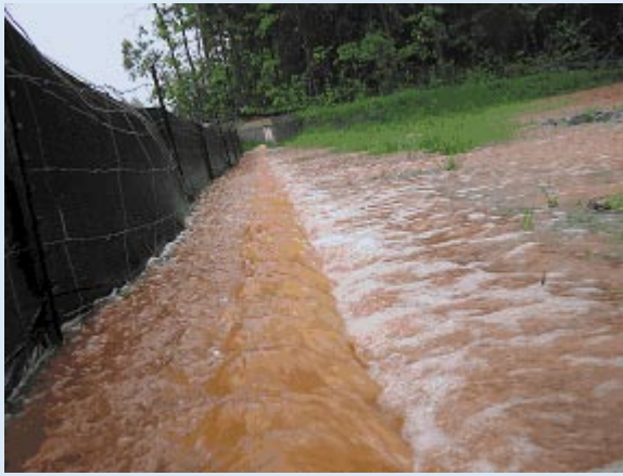
Figure 1. A level spreader providing diffuse flow (Frank Hahne, Mecklenburg County)
