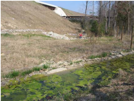
Figure 15: View of protected bank from back of level spreader
