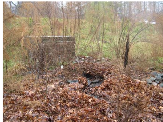
Figure 3: Level spreader approximately 3.5 years after construction
