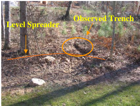
Figure 11: Earthen level spreader with channel
