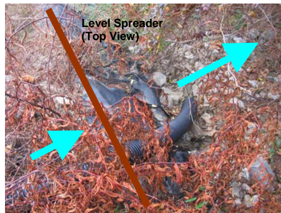
Figure 13: Drainage pipe laid over top of level spreader
