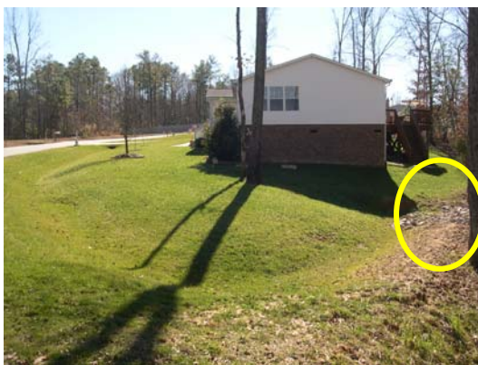
Figure 5: Swale leading to Level Spreader – Level Spreader Circled
