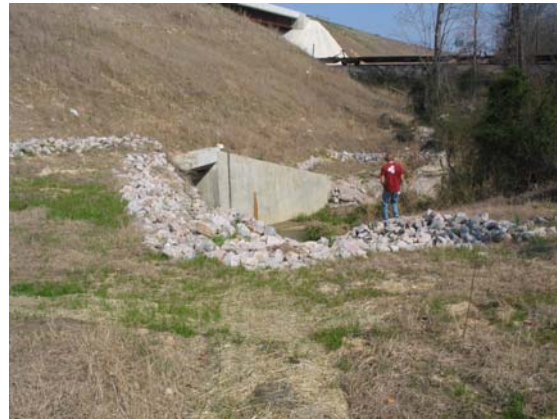
Figure 16: Close-up of protected bank
