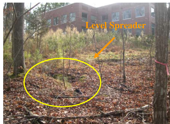
Figure 10: Natural swale downstream of level spreader (circled in yellow)
