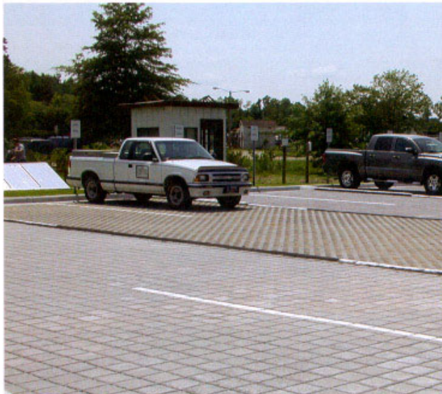
Figure 1. Runoff quantities and pollutants from asphalt and four permeable pavements are being evaluated by North Carolina State University in at a municipal-owned parking lot in Kinston, North Carolina.
