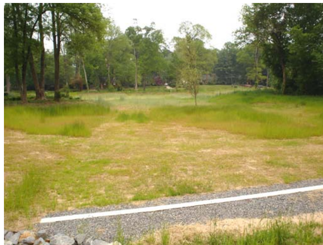
Figure 1: Filter strip down slope of level spreader.
