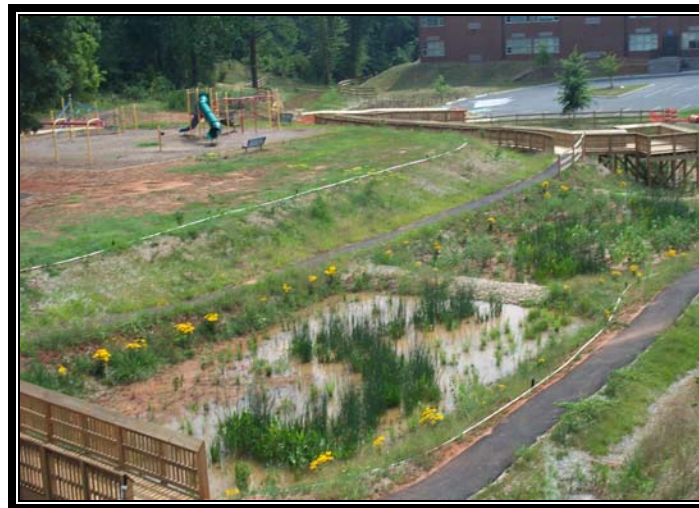
Figure 1. Bruns Ave. School Wetland, downstream view
