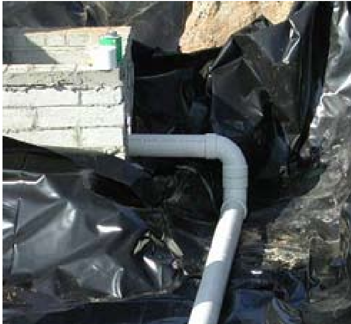
Figure 8. Installing a small upturn in the drawdown pipe will create an internal water storage (IWS) layer in a bioretention cell.
