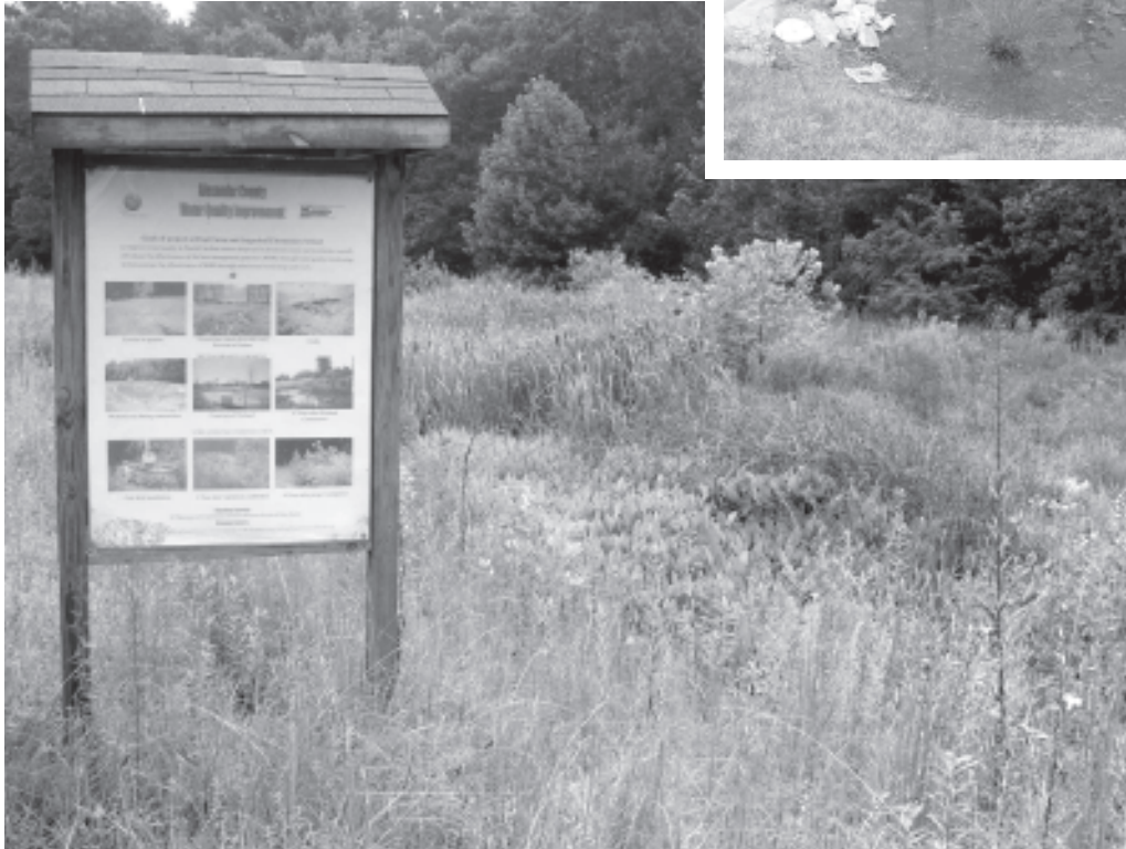
A stormwater wetland in Alexander County, heavily vegetated with wetland plants to filter rain runoff, is also an educational site.
