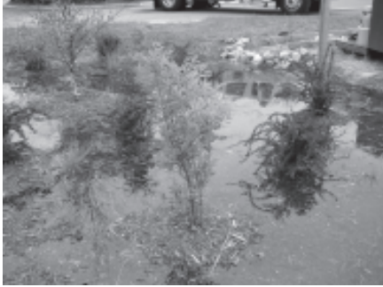
Two structural stormwater BMPs: a sand filter at NC State University (top) and a nearly full bioretention/raingarden in Chapel Hill.
