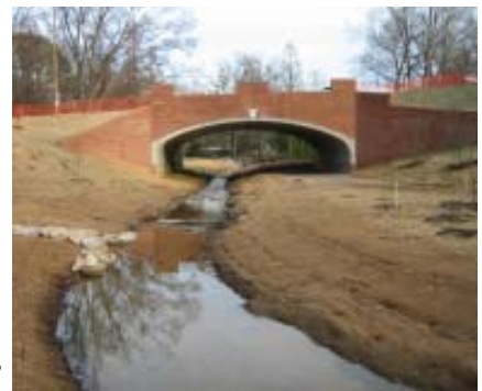
Pullen Rd. Arch Culvert
