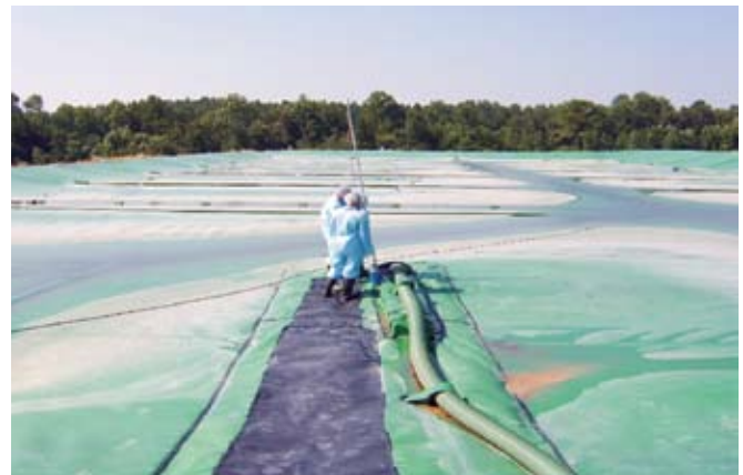
Figure 2. Covered lagoon at Black Farms near Lillington, N.C. Cover was installed in 2008. Cover has ports for recycle lines for flush water and irrigation pump intake as well as a pipe system across bottom of lagoon for removing sludge. Two lagoons for 6000 finishing pigs were covered.
