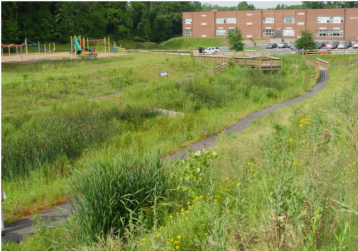
Bruns Elementary School stormwater wetland: Wilmington, NC.
