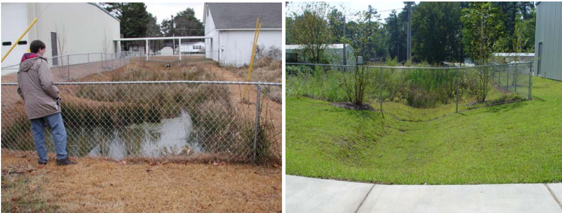
Figure 13. Spring Lake VFD Pocket Wetland. Left view is from the rear of the wetland in the winter. Right view is the front of the small wetland in early fall.
