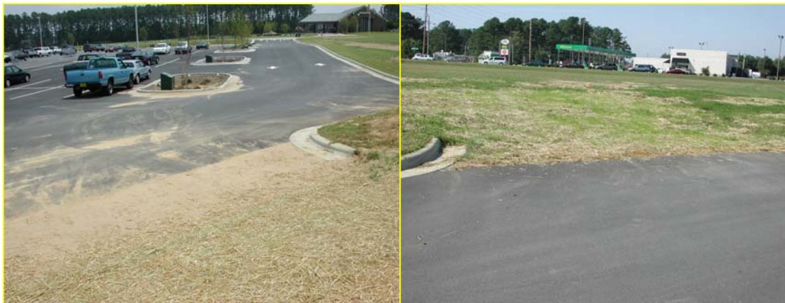
Figure 10. The watershed remained unstable for several months. Sediment from the unstable areas found its way into two of the basins, as seen in the picture to the left. The entranceway was seeded and reseeded throughout the summer and fall of 2002. By November and December of 2002, the entranceway was deemed stable.
