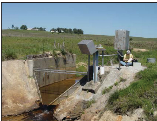
A view of one of the projects paired watersheds. The H-Flume with instrumentation records flow rates and samples for water quality.
