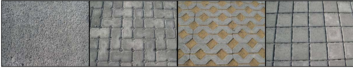
Figure 2. Permeable pavement sections surfaced with (left to right) pervious concrete, permeable interlocking concrete pavers with 12.9% open surface area (PICP1), concrete grid pavers, and permeable interlocking concrete pavers with 8.5% open surface area (PICP2).
