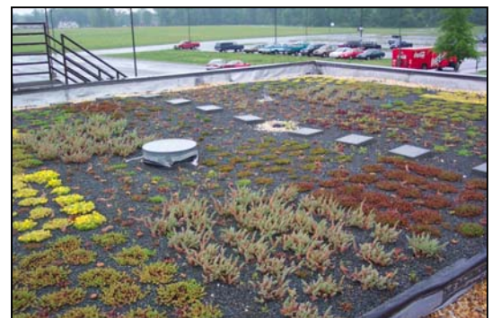
Figure 3. WCC Greenroof in Goldsboro (April 2003).
