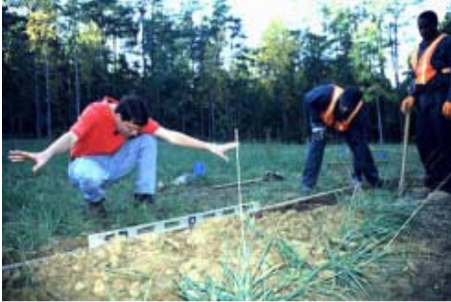
Figure 3. Installing a Pretreated Lumber Level Spreader
