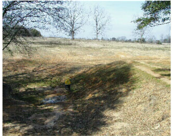
Figure 5. 4-S watershed critical area one after BMP installation (sediment reduction structure).
