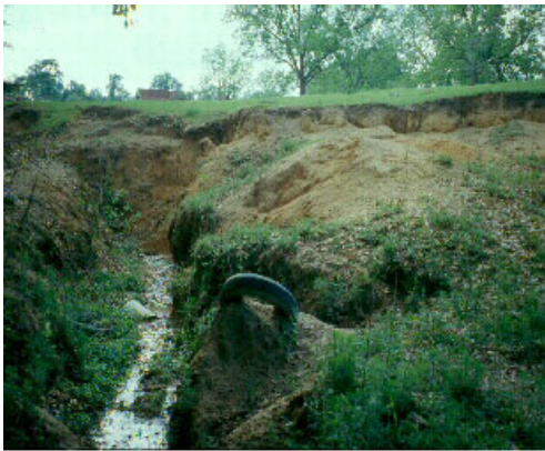
Figure 4. 4-S watershed critical area one before BMP installation.
