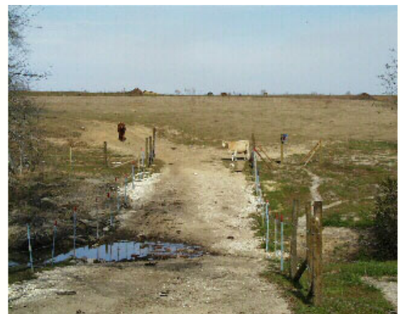
Figure 6. 4-S watershed constructed cattle crossing.
