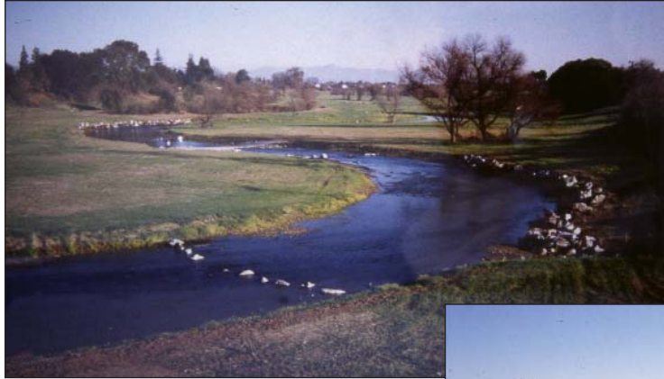
Errors on trial. Rosgen’s ideas have inspired expensive failures, critics say, such as engineered meanders on California’s Uvas Creek (above) that were soon destroyed by floods.
